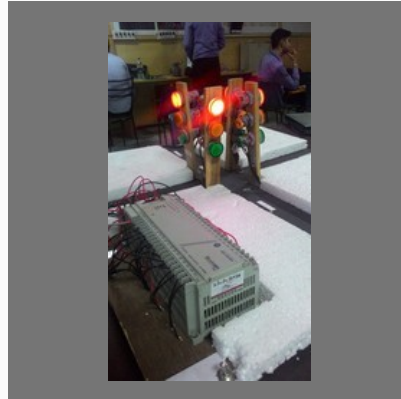
PLC Based Traffic Light System
